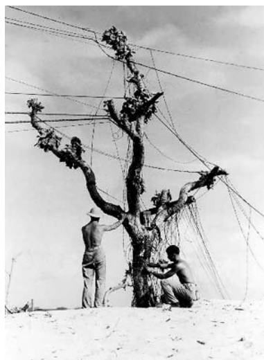
Communications Men string telephone wire onto a tree, US Department of Defense
